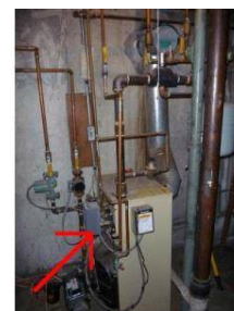
Wtr tmp, tankless coil, no TP valve.
