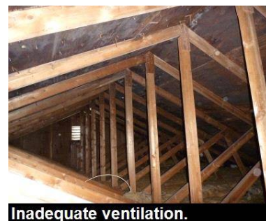
Inadequate ventilation.
