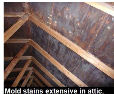
Mold stains extensive in attic.
