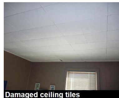
Damaged ceiling tiles
